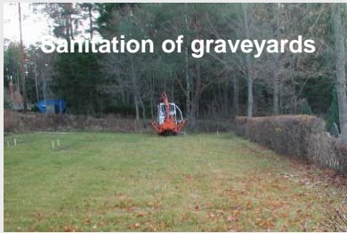
(Fig. 2a) For an efficient sanitation it is important, to define the exact position of the graveyards .
