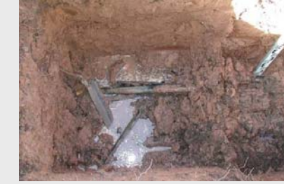
(Fig. 2c) By opening some of the graveyards during the sanitation it showed that the georadar displayed the correct positions.
